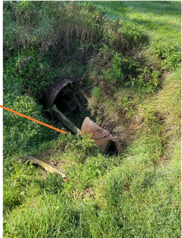
Wood cribbing is failing
