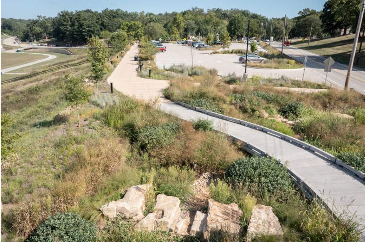
Green parking lot with perimeter bioswales and rain gardens in South Park.
