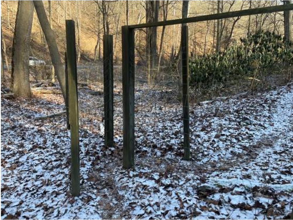
Zig-zag fence opening at Trillium Trail wildflower reserve. Pedestrians can pass freely with no gate, but deer are excluded. Overhead diagram of fencing: ---< ----
