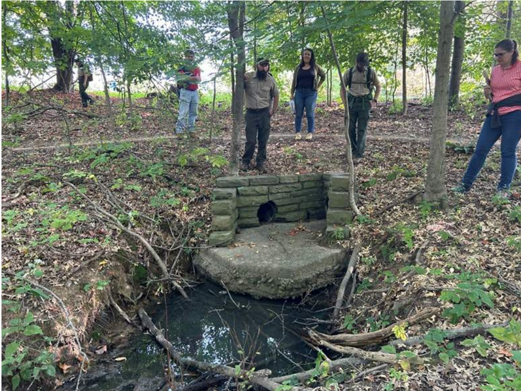
Culvert outfall in nearby forest.
