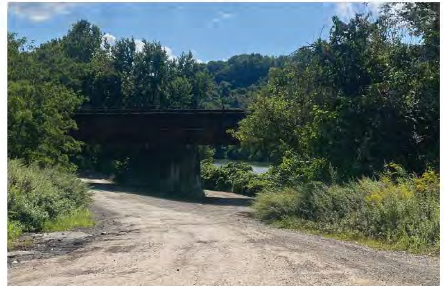
P & LE BRIDGE NEAR THE EXISTING DOUGLAS STREET TRAILHEAD
