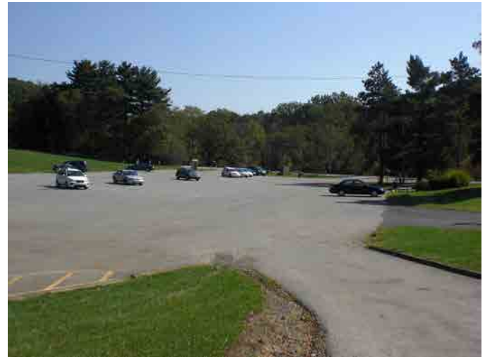
existing parking lot with large expanses of impervious paving that enables stormwater to pollute the lake and streams
