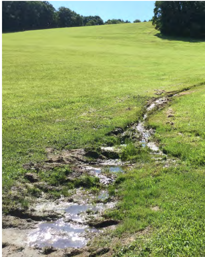
Erosion in Field into Middle Road - MGMT Zone 1
