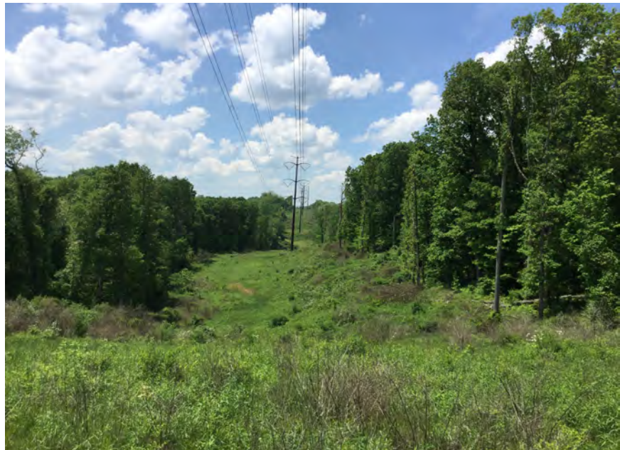
Utility Right-of-Way in Management Zone 1, West of the Pond
