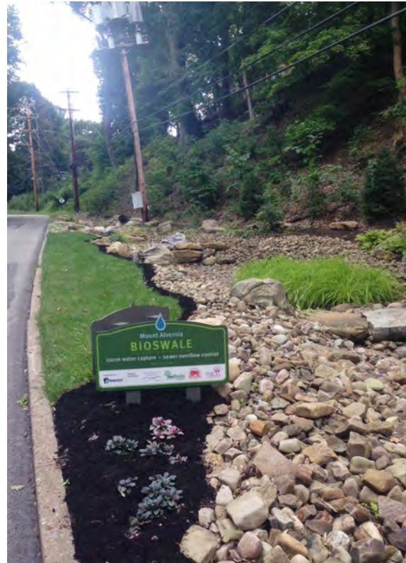
Bioswale and its signage along Hawthorne Road in Millvale, PA.
